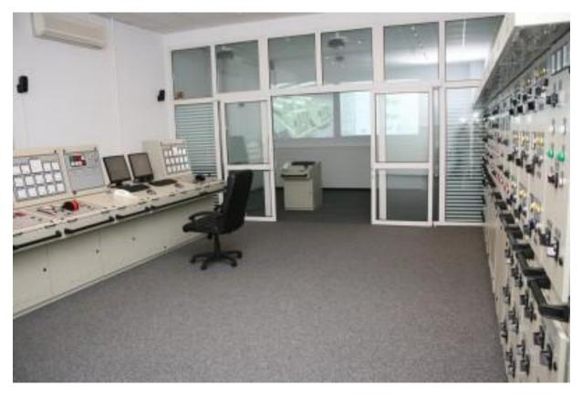
The UNITEST full mission engine room simulator is based on very modern solutions, which are presently used in medium-sized, computer-controlled engine rooms. The engine room simulator can operate with two (2) models of propulsion plants: a medium speed (one four-stroke type main engine with reduction gear and controllable pitch propeller) and a low speed (one two-stroke type main engine with fixed pitch propeller).
