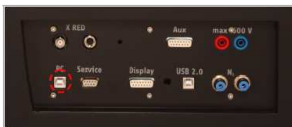
Fig. 4: Connection of the computer
